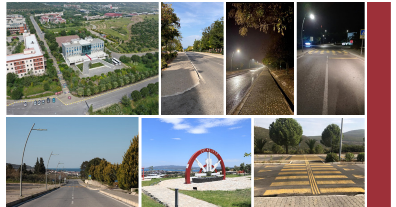
Figure 10: At IZTECH, all sidewalks are lightened and separated from the roads by elevation. The sidewalks are designed as accessible for physically disabled persons. All crosswalks are marked with pavement markings and traffic signs. The elevated crosswalks are used as speed ramps for speed limit enforcement especially where the pedestrian traffic is high.
