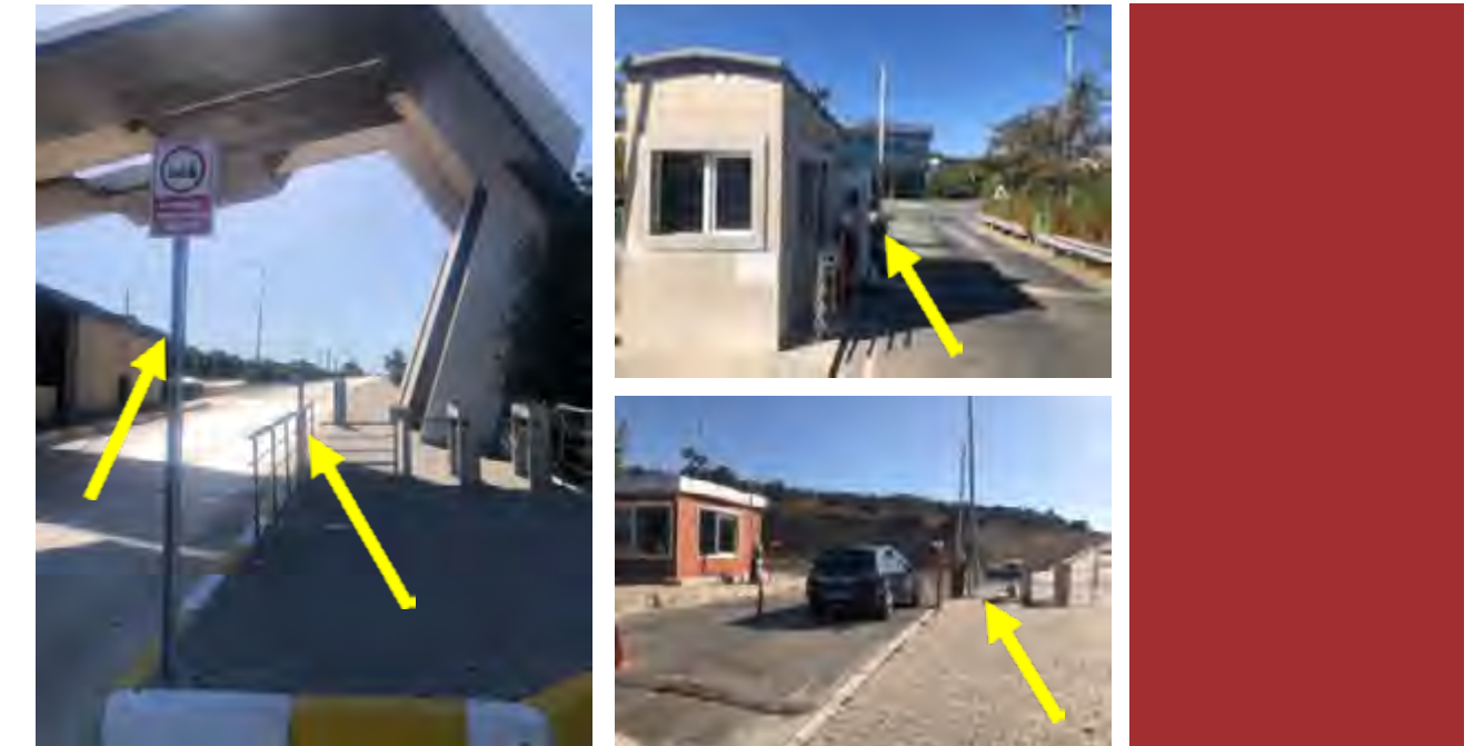
Figure 1. License-Plate Recognition Systems (LPRS) located at each gate
