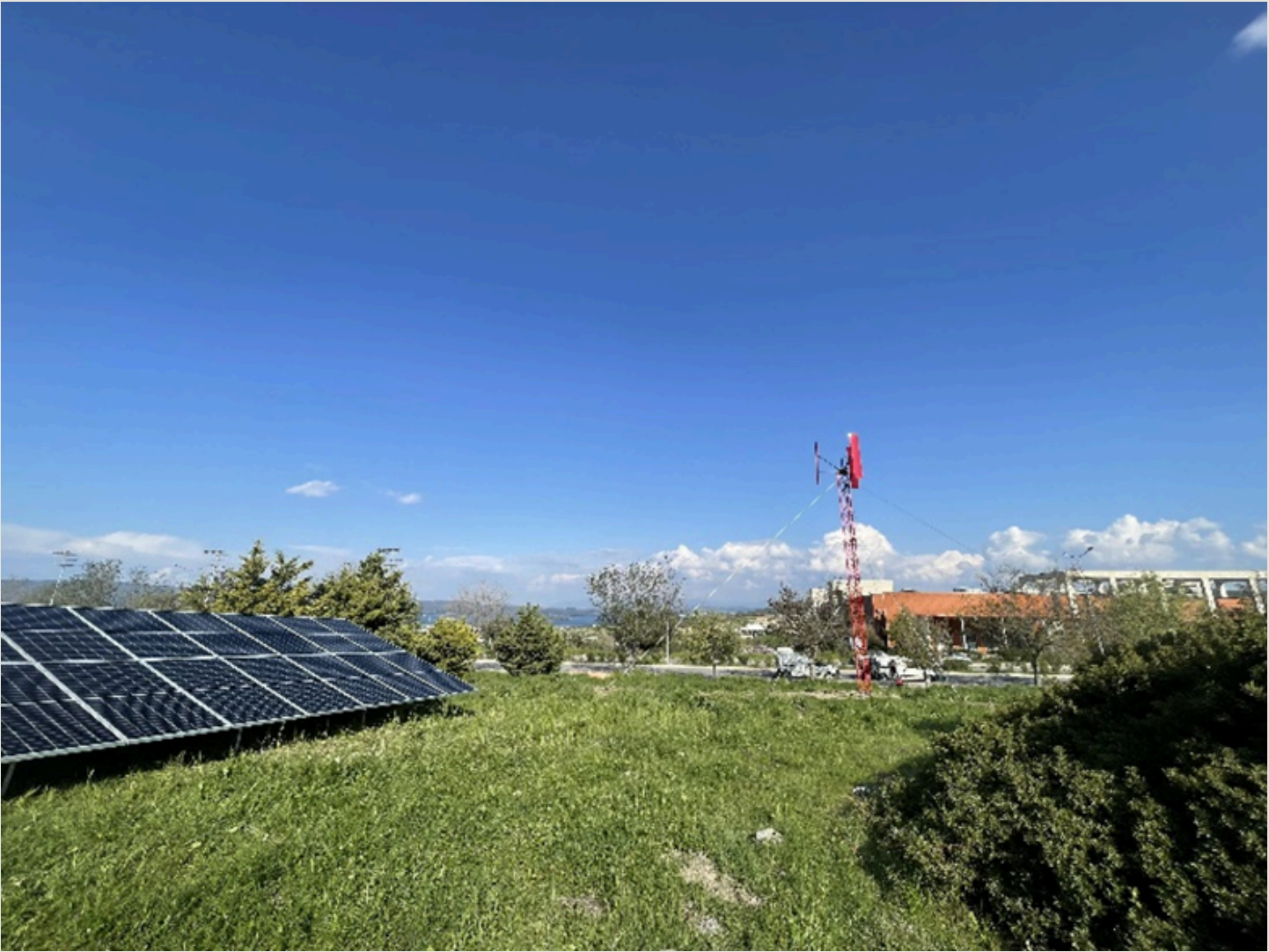
Figure 5: The vertical axis wind turbine used in the project
